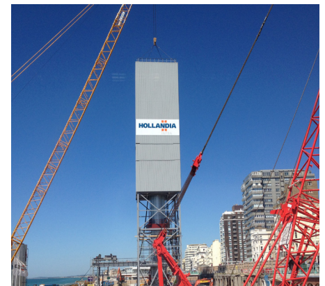
The jacking tower in place
